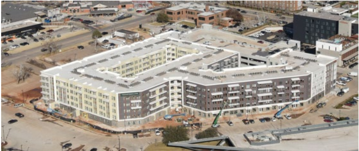
6161 N Western Ave., Oklahoma City, OK (Pre-Fire Photo)
